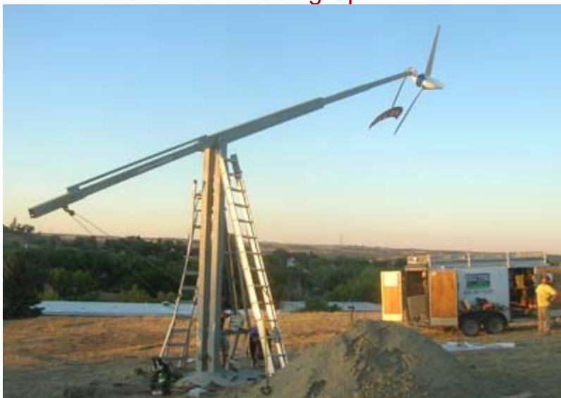
The first of three wind power generators has been installed on the hill by the N. The electrical power inverter and auxiliary net-metering equipment are located in the Automotive Diagnostic Building. The wind power generator is an ARE 110 made by Abundant Renewable Energy Inc. The wind power generator is a 2.5 KW system that will produce approximately 340 KW hours of energy a month; which is about enough to power a normal home for the month.
